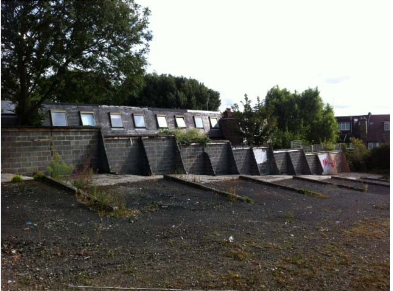
Northern Boundary Wall of Site
